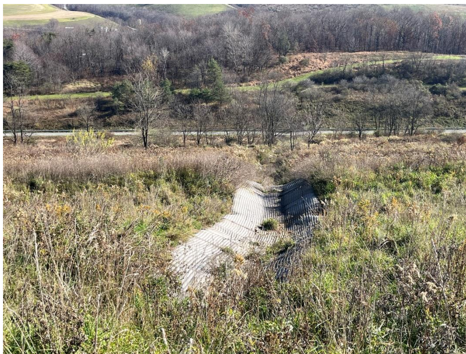
Photograph 21. East Valley Slope Drain, view east from Stage III top.
