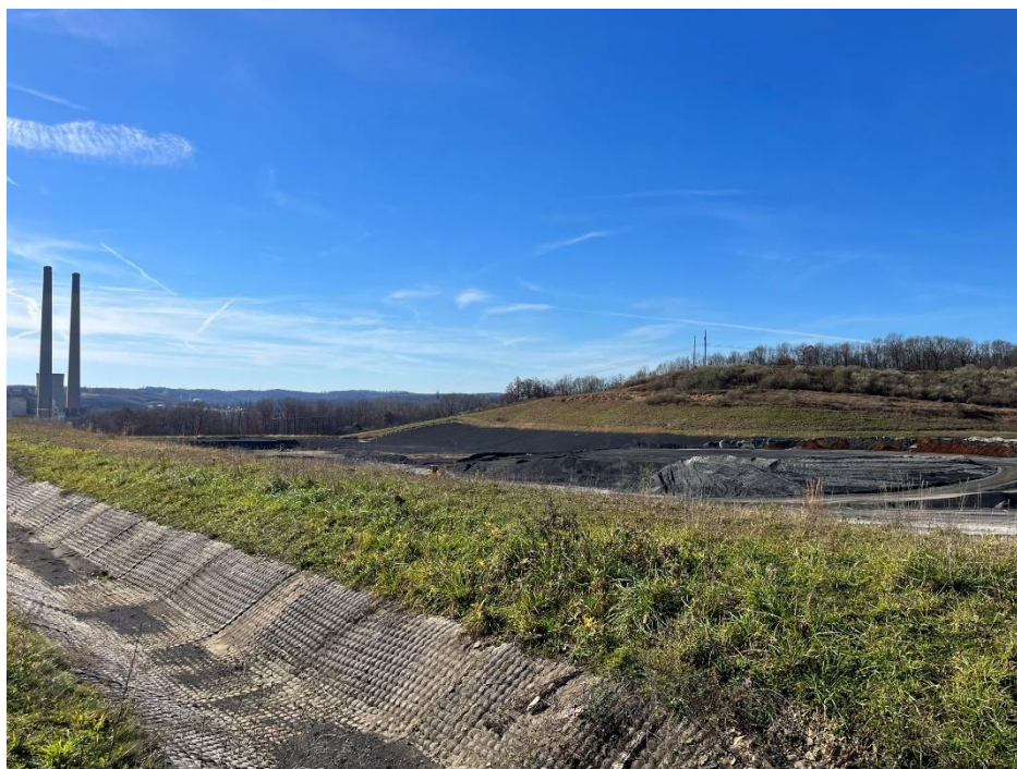
Photograph 26. West Valley Stage IV and haul road collection channel, view south.
