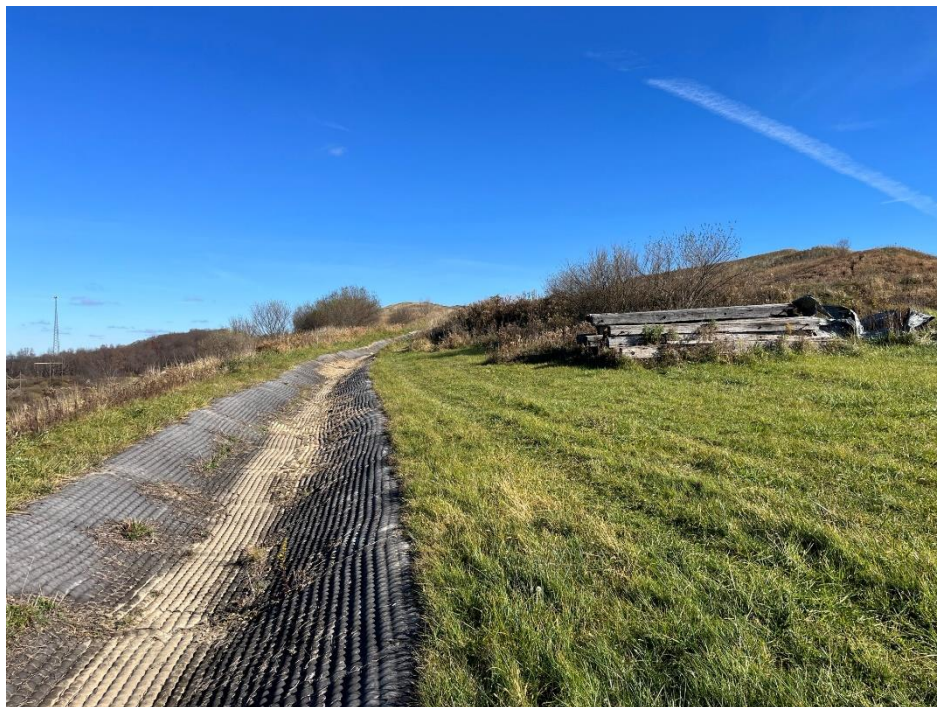
Photograph 16. West Valley Stage III Diversion Channel, view north.
