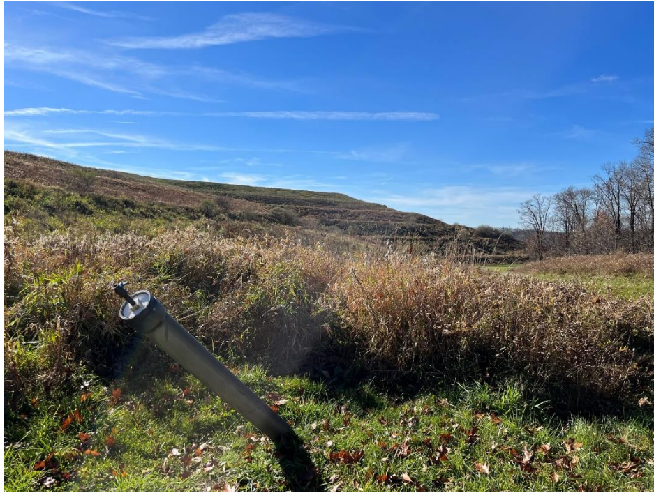
Photograph 15. Foreground – Stage 1 west facing benches and leachate pipe cleanout. Background – Stage III west facing benches.
