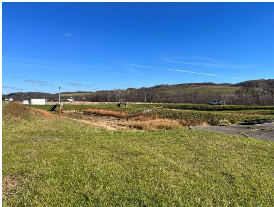
Photograph 9. View north of idled East Valley Equalization Ponds.
