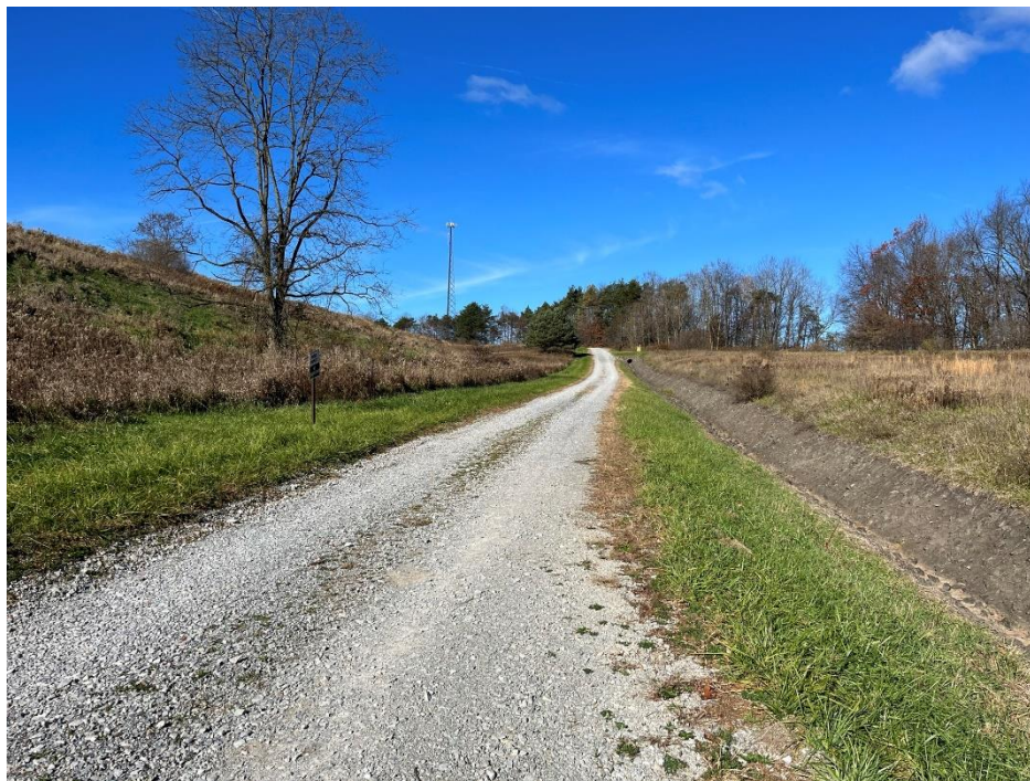
Photograph 13. East Valley east facing benches and Stage I/II collection channel, view north.
