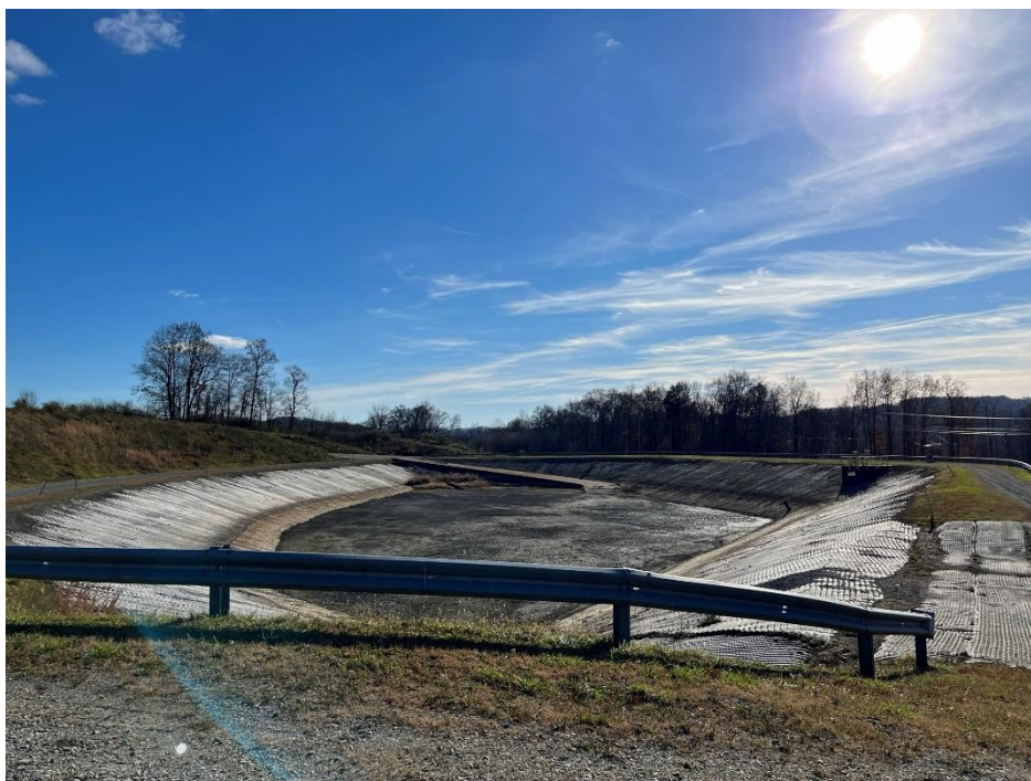
Photograph 2. West Valley Equalization Pond, view southwest.
