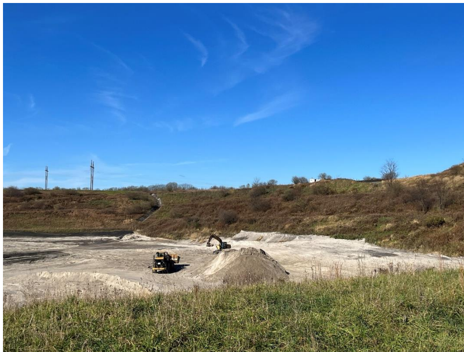
Photograph 25. Gypsum being loaded out of a stockpile in Stage IV for beneficial use.
