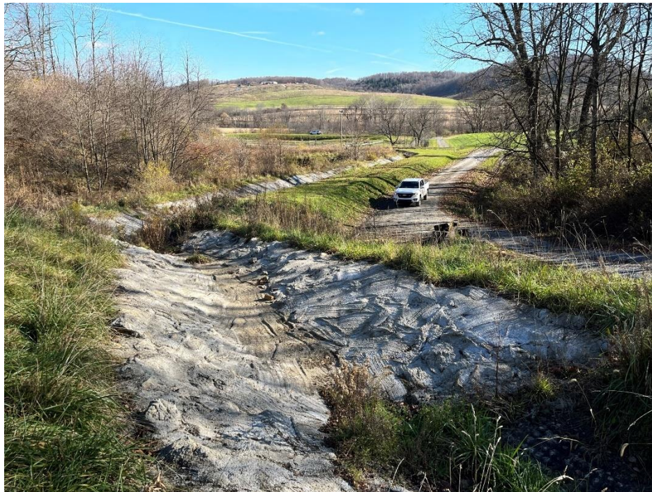
Photograph 6. East Valley Collection Channel at toe area, view east.
