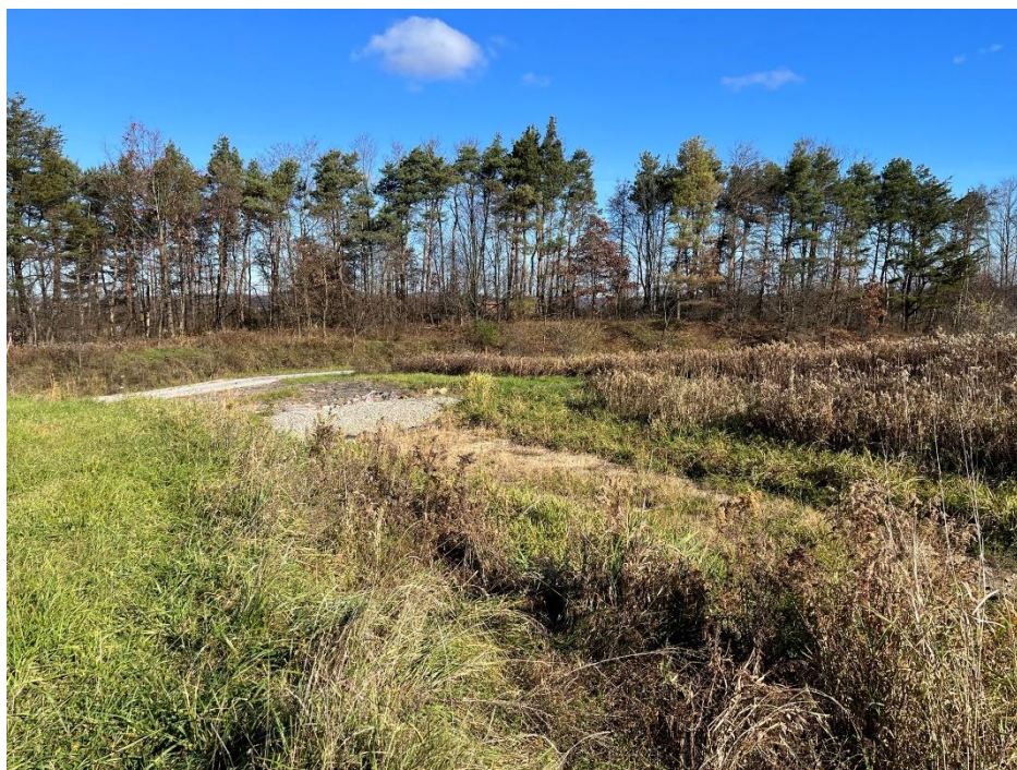
Photograph 14. Stage I/II revegetated top surface drainage swale, north end.
