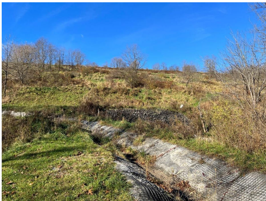
Photograph 8. East Valley Toe and east facing benches, view west.
