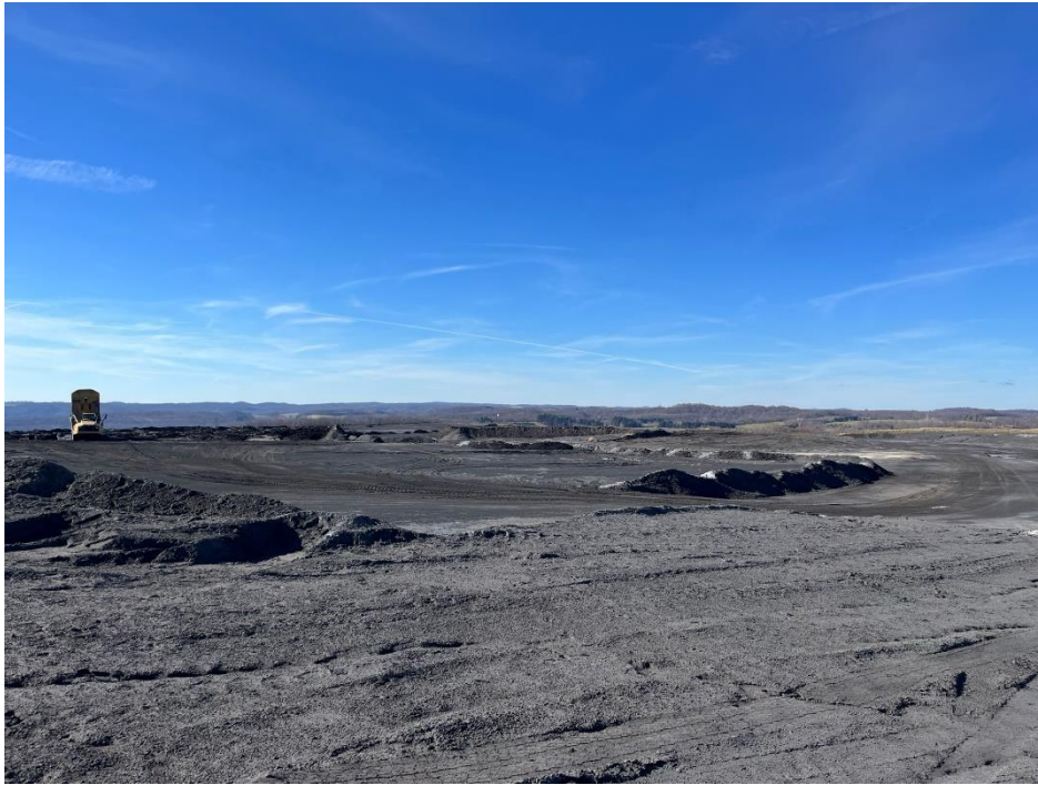
Photograph 23. Active top of West Valley Stage III.
