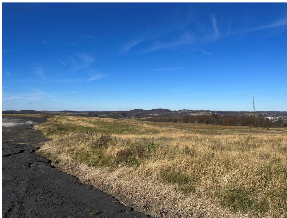
Photograph 22. North end of revegetated Stage III top.
