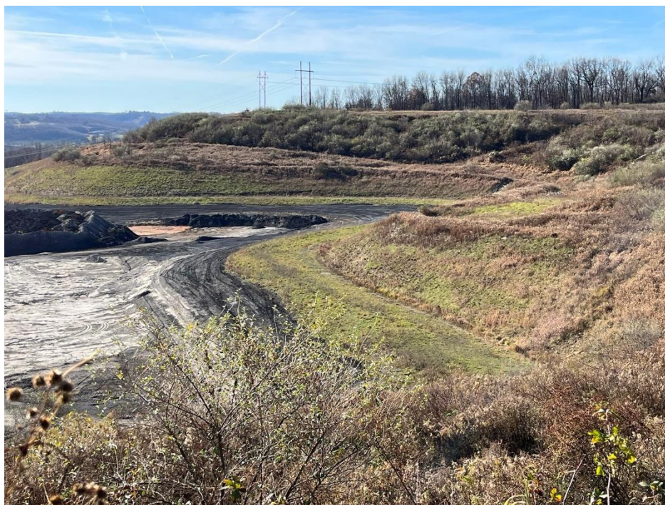
Photograph 18. West Valley Stage IV, view southwest.
