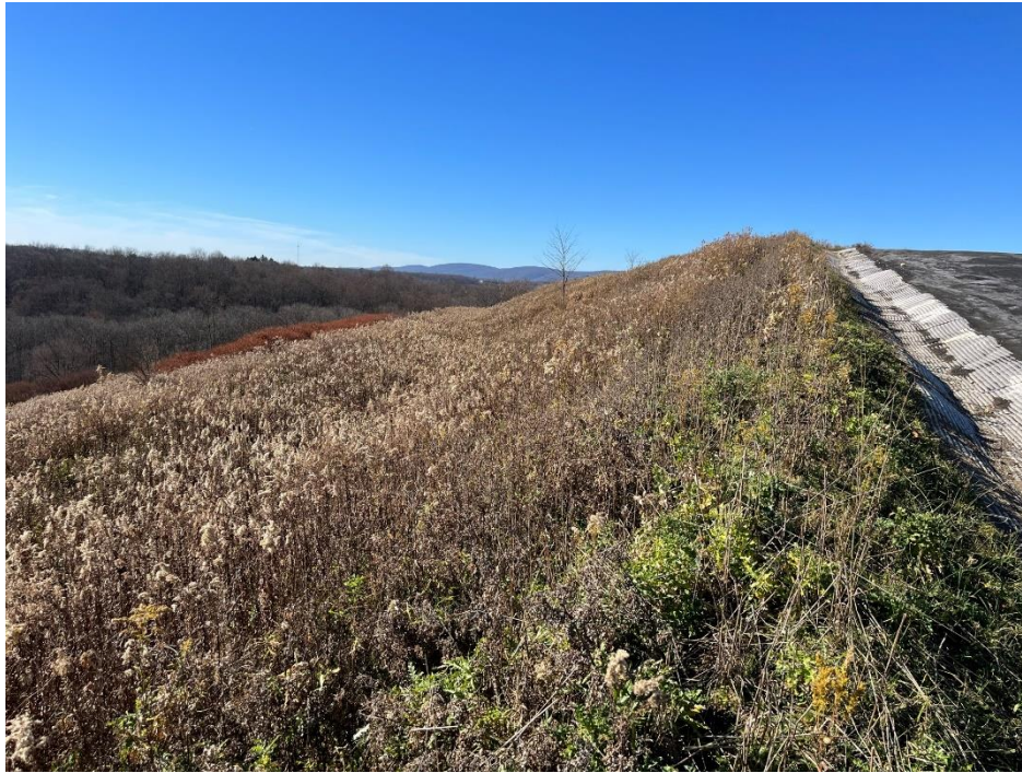
Photograph 19. Southern slope benches of Stage II; view west.
