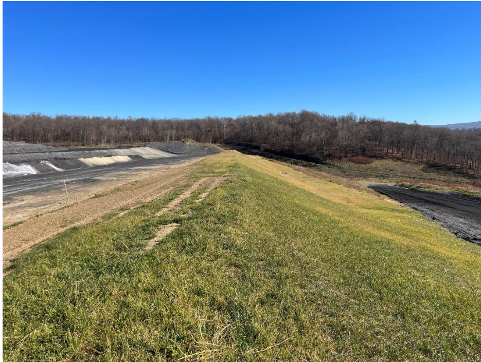
Photograph 17. Southern benches of Stage II, view east.
