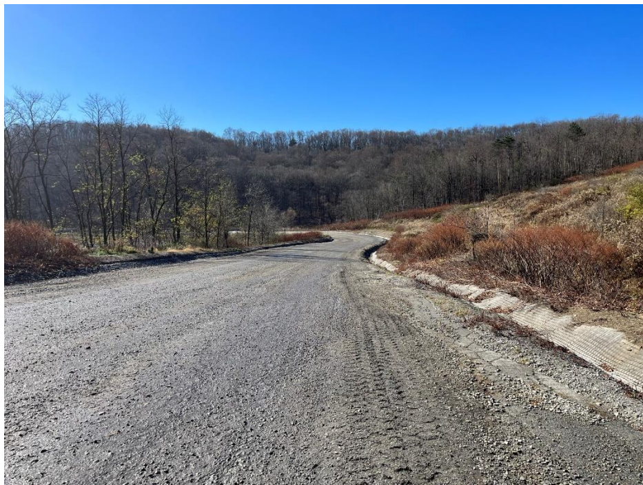
Photograph 21. Haul road with Stage II benches (right); view west.
