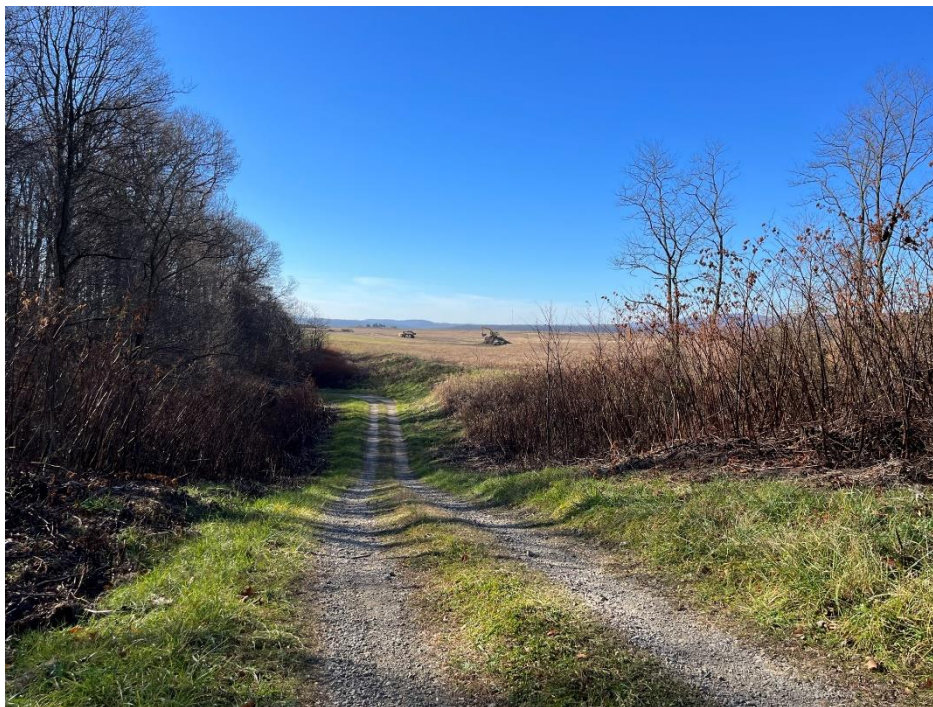
Photograph 11. The vegetated northeastern side of Stage II (foreground) and active Stage II in background; view southwest.
