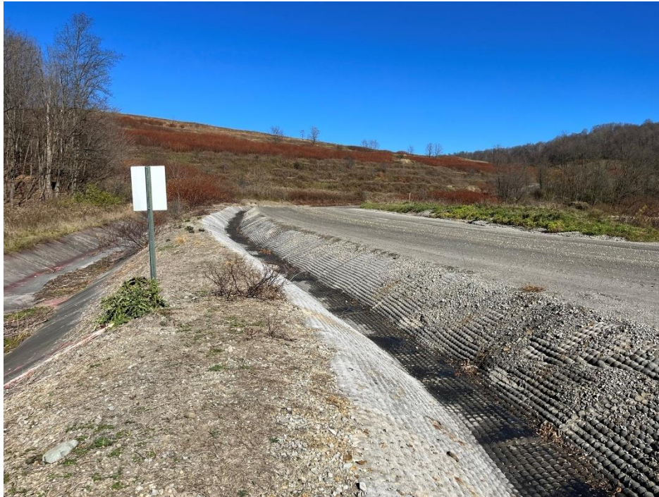
Photograph 23. Channels and revetment along the Stage II haul road; view northeast.
