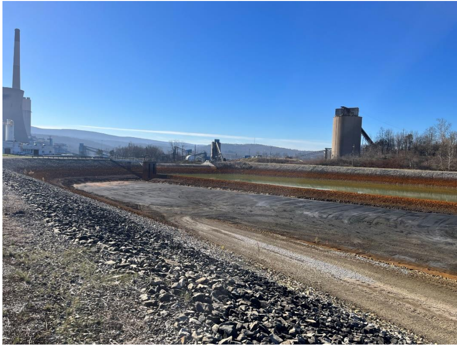
Photograph 1. Equalization Pond, immediately north of disposal site treatment plant; view southeast.
