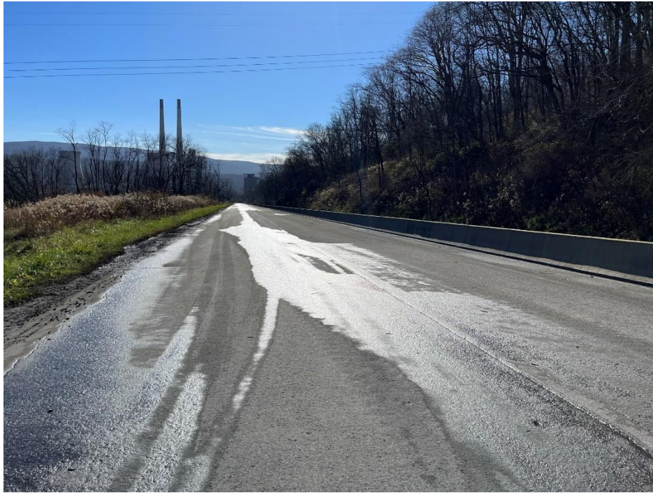
Photograph 25. Haul road south of Stage IIIA ; view south.
