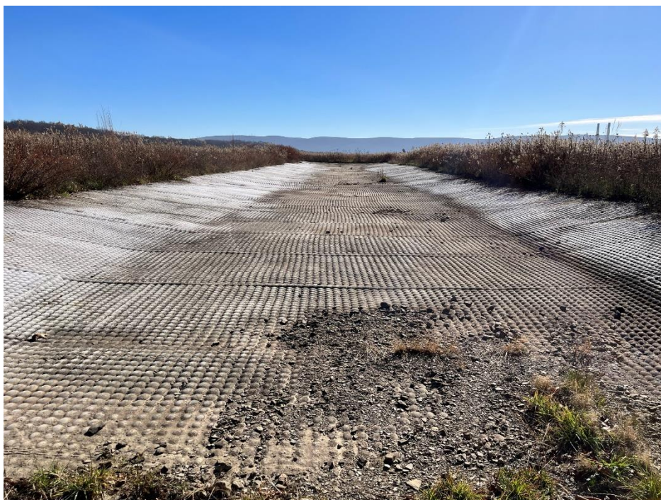
Photograph 12. Stage II northwest top surface drainage channel; view southeast.
